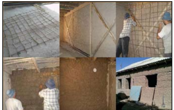
Workers build an earthquake-resistant home with "mulberry branch technology"
